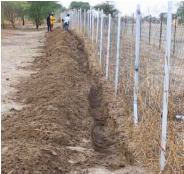
Picture: Sand removal works carried out along the perimeter fence. Sand accumulation against the fence reduces its effective height, posing a significant risk to the safety and containment of the ostriches. Date: June 2025
