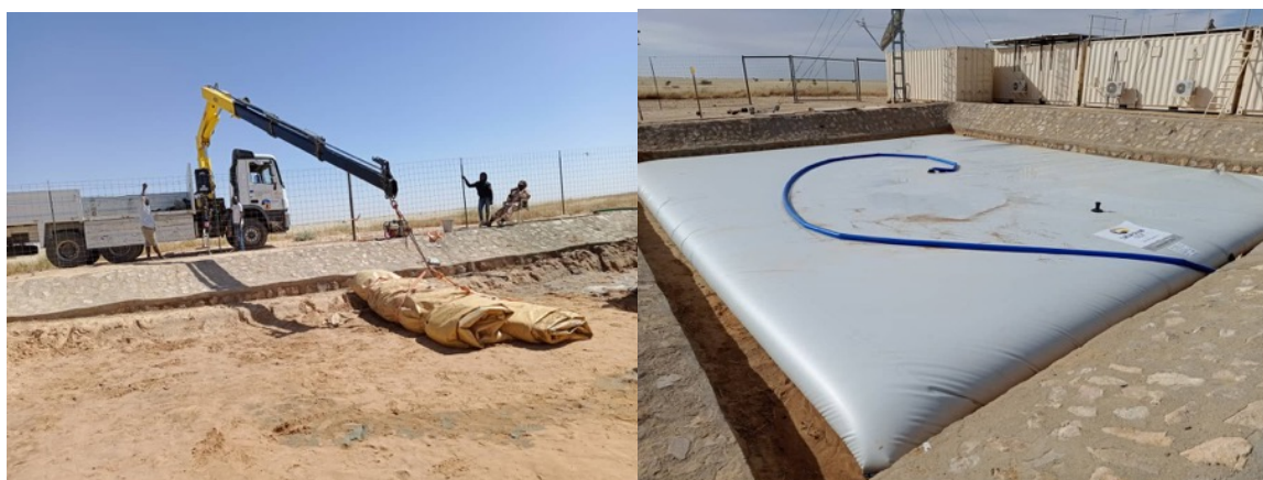
Fig. 5. Installation of the new water tanks.
