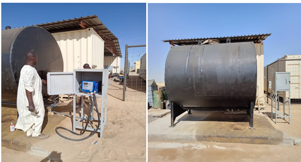
Fig. 8. New diesel tank on slab and base + pump
